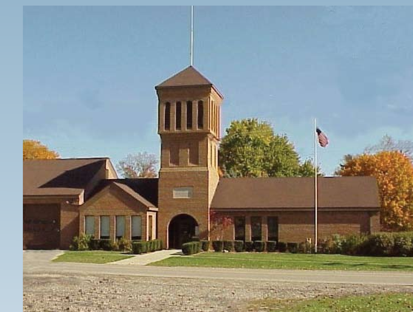
Government Services Manchester Township Hall
